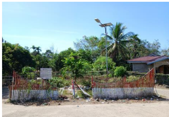
Figure 1. The Condition of the Park Before Renovation
