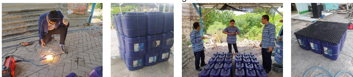
Picture 5. Frame Welding Process, Jerry Can Assembly for Pontoon, Pontoon with Frame, Addition of Drainage Cell as Deck
