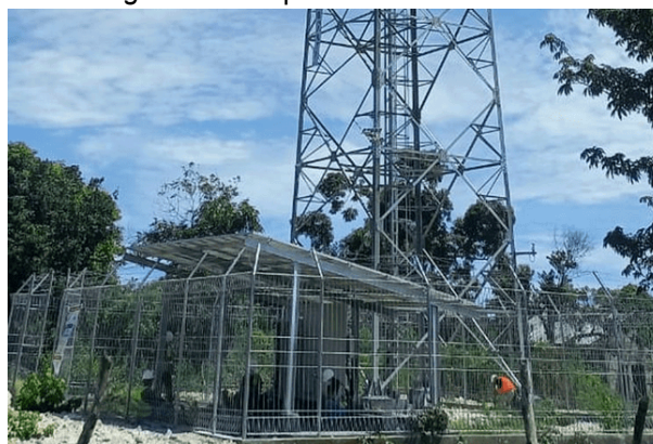
Figure 2. Adequate Internet Facilities
