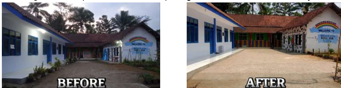
Figure 7. The prior and after block paving installation on school's front yard.
