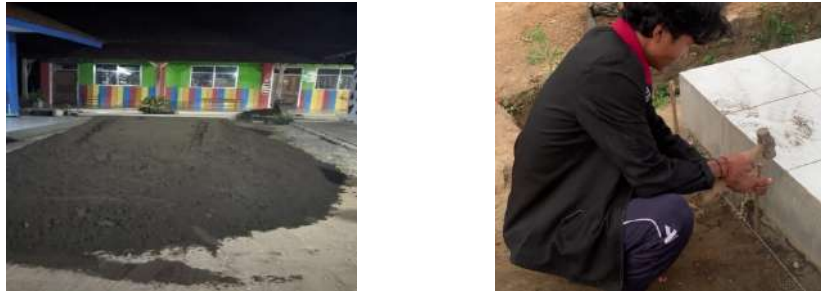
Figure 5. Installation of paving block.
