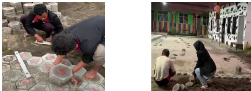
Figure 6. Installation of edge concrete restraint.
