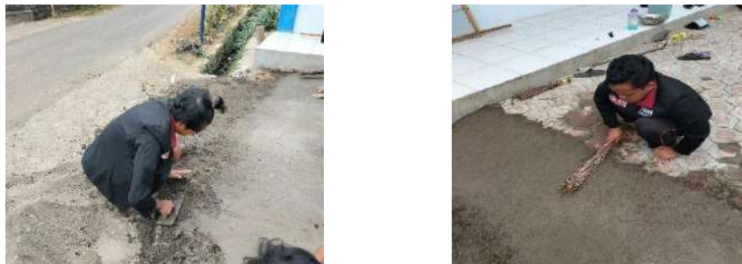
Figure 6. Installation of edge concrete restraint.
