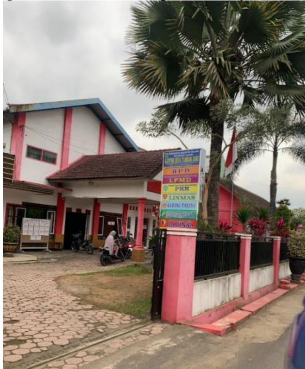
Figure 2. Tambakasri Village Office, Tajinan District
