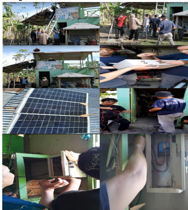
Figure 4. Installation of Solar Panel Installation
