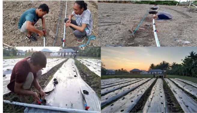
Figure 5. Installation of Drip Irrigation System
