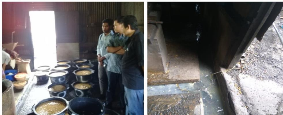
Figure 2. Waste disposal system of a tofu factory
