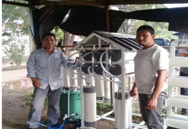
Figure 4. Installation of a waste treatment plant at the SOLO Tofu Factory
