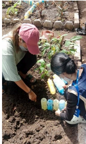
Figure 2. Construction of Borders and Soil Retainers
