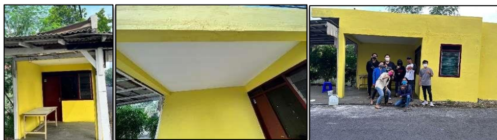
Figure 11. Results of the renovation of RT 04 Wisma Permai Guardhouse
