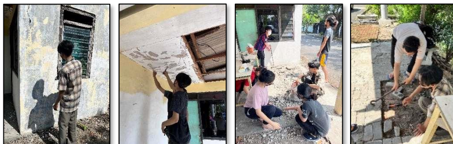
Figure 8. From Left: Wall Cleaning; Ceiling Dismantling; Floor Dismantling; Paving Block Dismantling
