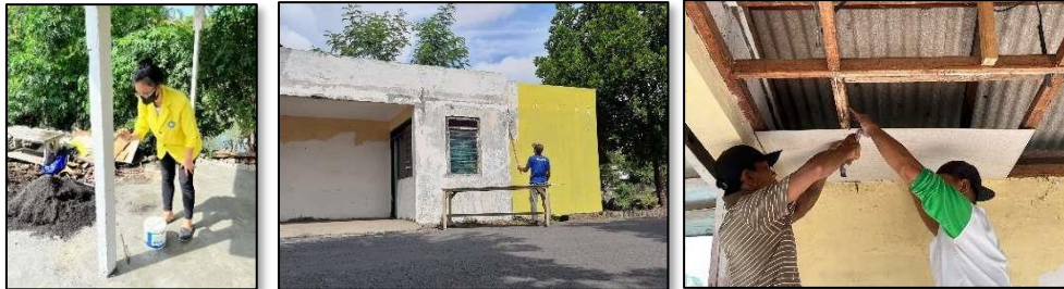
Figure 9. From Left: Wall Painting; Ceiling Installation
